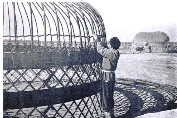
Fig. 2. The tent frame during erection, the shepherd is fastening the struts with a duz yup . Atabay Yomut. [Image archive of Tarbiat Modares University]
