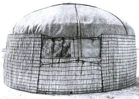
Fig.1. Aq oy, from the back, showing felt junctions. [Image archive of Tarbiat Modares University]
