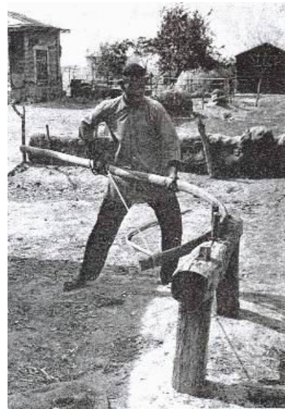
Fig. 8. Manufacture: bending a felloe for the roof ring. Ceperbay Yomut [Image archive of Tarbiat Modares University]
